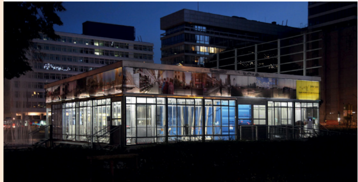
The BHRÖX bauhaus reuse, constructed out of former windows of the famous Bauhaus Dessau, transformed into an open-air exhibition at Ernst-Reuter-Platz, Berlin (© Janin Walter).
