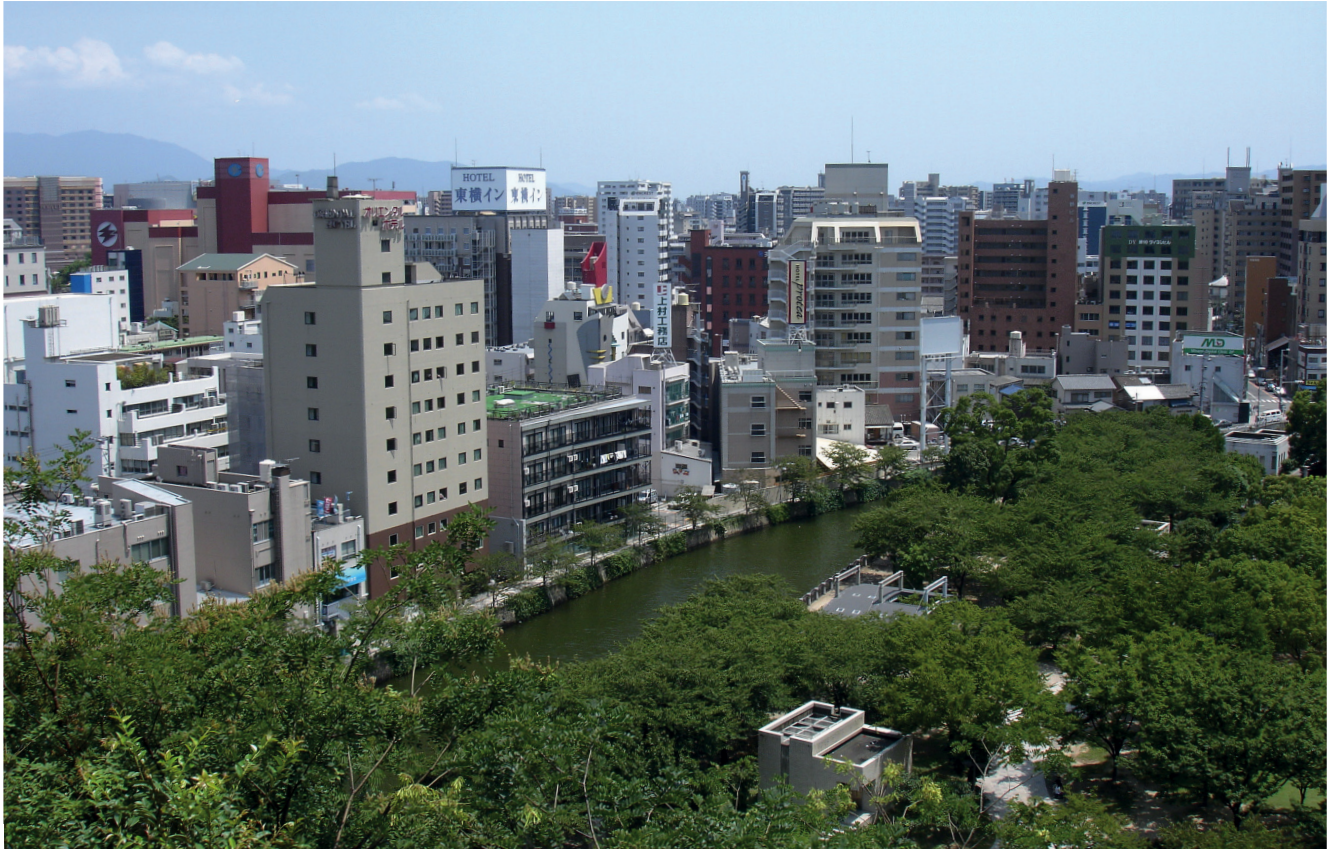
Tenjin, Fukuoka's most dense neighborhood, seen from the green roof of the ACROS building, the symbol of the city's heat adaptation plans (© Wikimedia Commons).
