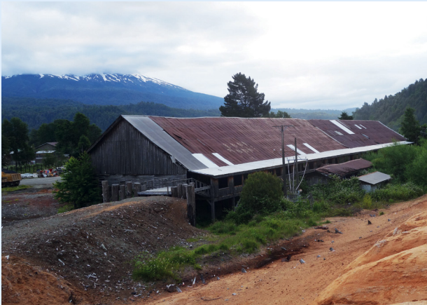
Out of use: The old wood factory in the center of the village with the "cerro de aserrín", a mountain of wood chips from the last 100 years (© Jae-Young Lee).
